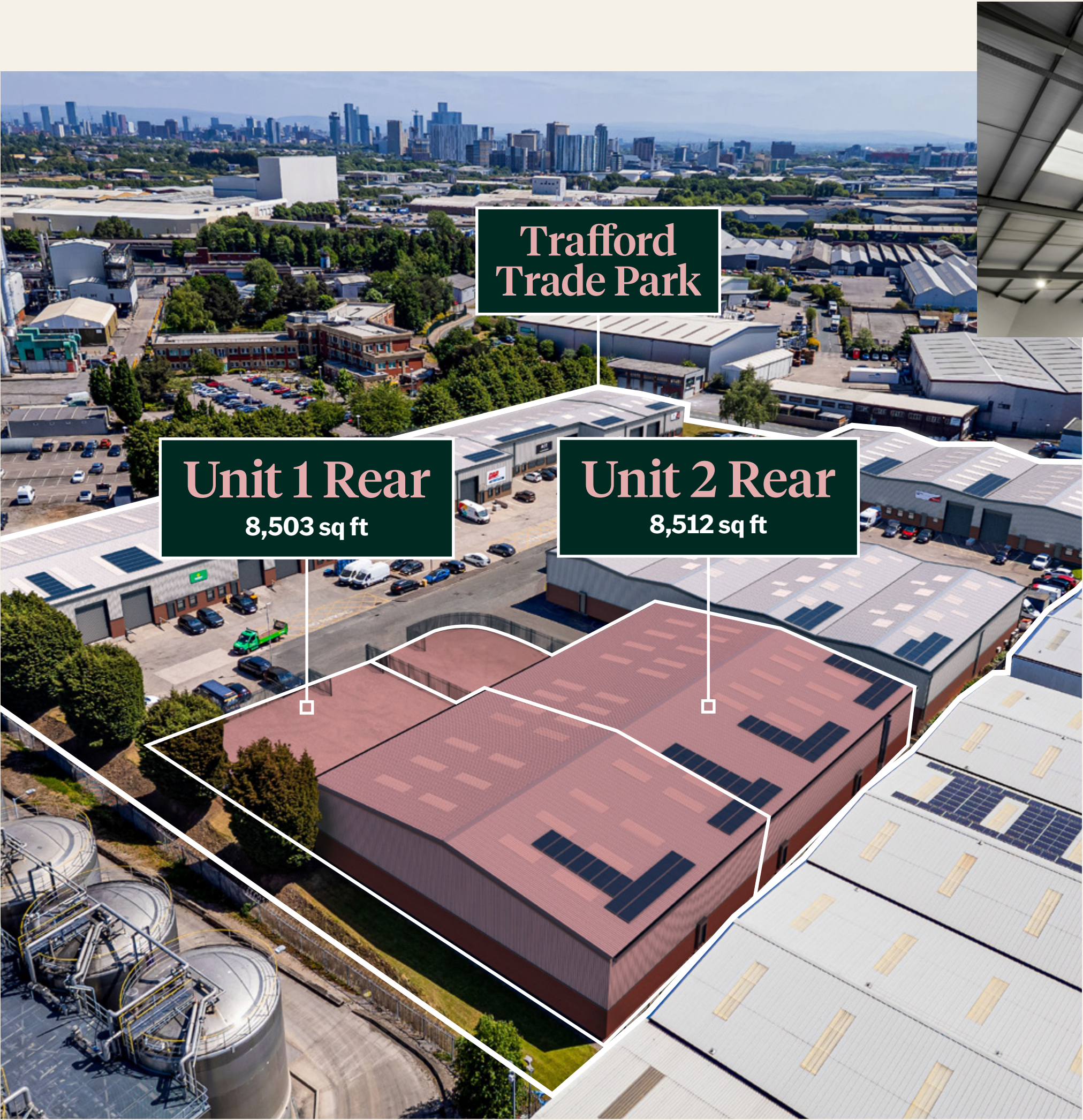
• Computer generated image of Units 1 & Unit 2 Rear
