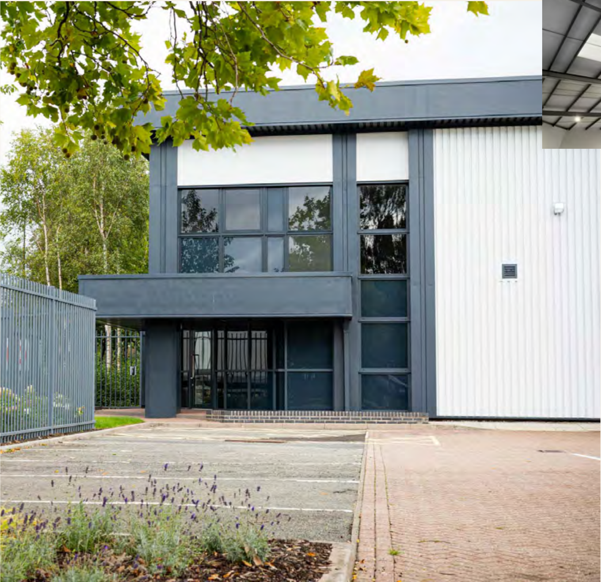
• Unit A Exterior
